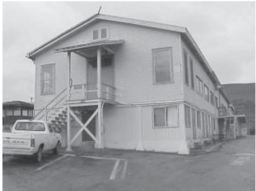
Figure 31. Original Wilson Cove Messhall & Chapel - Bldg. 60103 (1936-1999).
